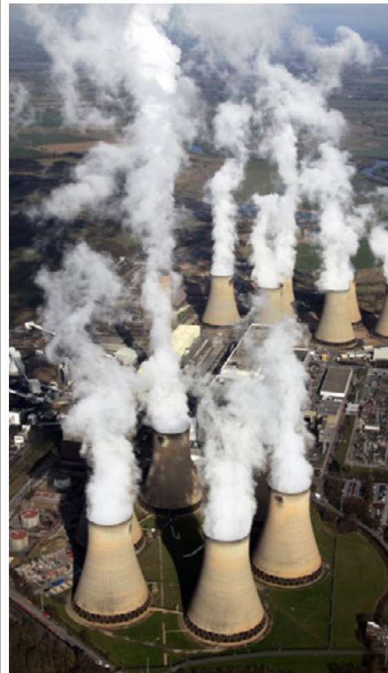
Drax Power Station
